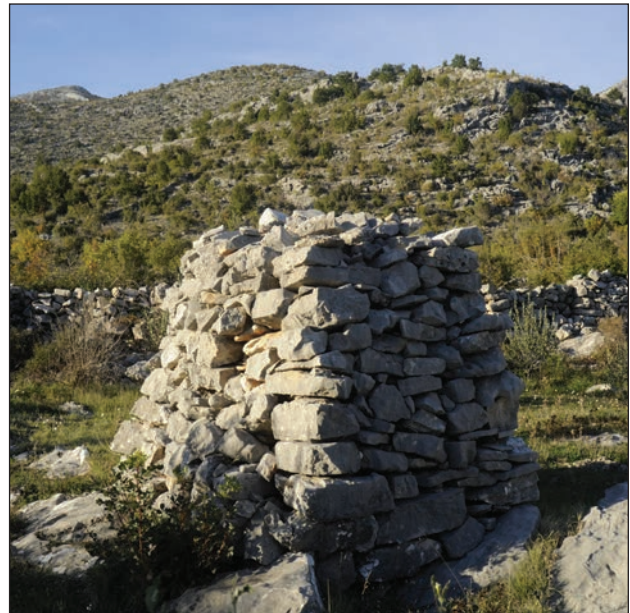
Figure 8: Freestanding constructions for depositing stones from a pasture can be seen in a wall in Herzegovina near a ‘poljarica’ (Freudenreich) (Photo: B. Juvanec).
