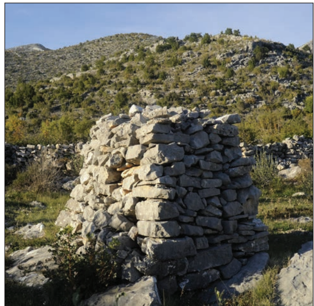
Figure 8: Freestanding constructions for depositing stones from a pasture can be seen in a wall in Herzegovina near a ‘poljarica’ (Freudenreich) (Photo: B. Juvanec).
