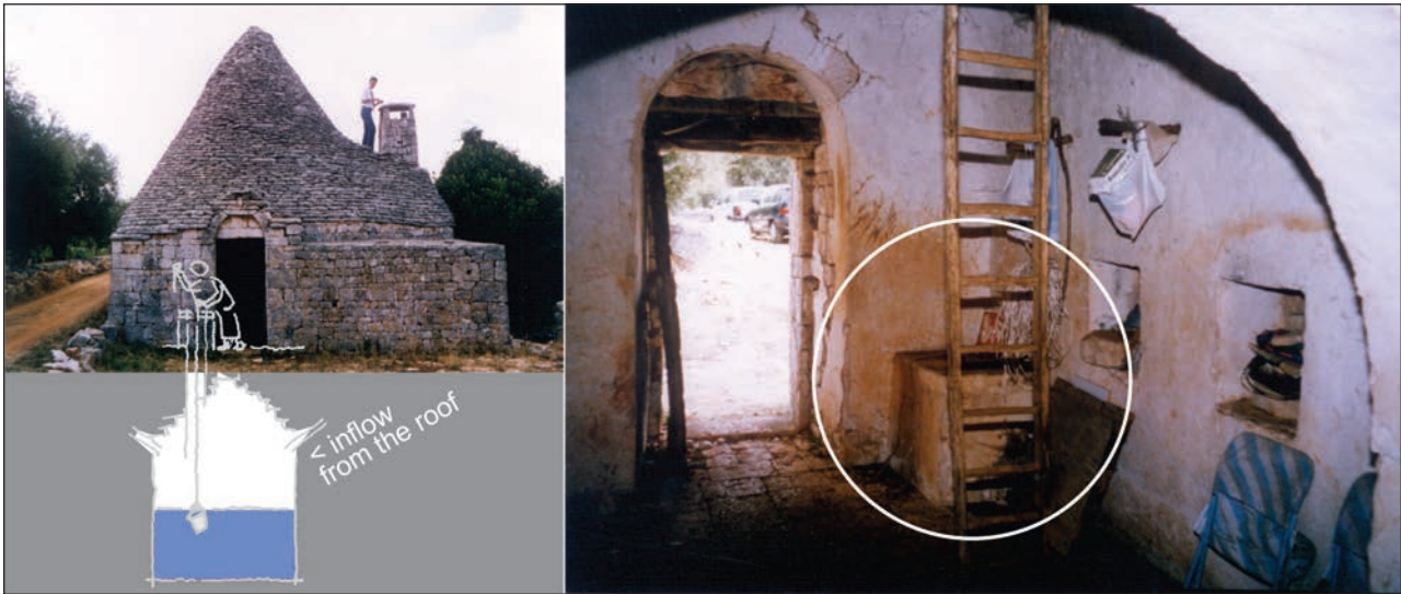
Figure 15: The reservoir is cut into the ground under the kitchen. Water is collected from the roof of the living and auxiliary parts of the homestead in Puglia (Masseria Maccherone near Alberobello) (Photo: B. Juvanec).
