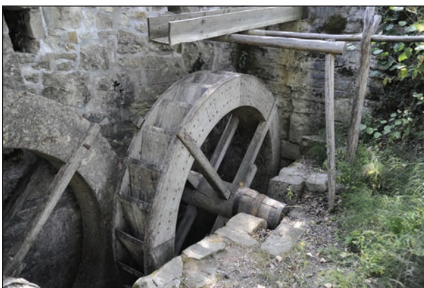
Figure 16: The construction of the milling system is all in wood, while the building construction is all in drystone (Mazurin's watermill in Slovene Istra) (Photo: B. Juvanec).
