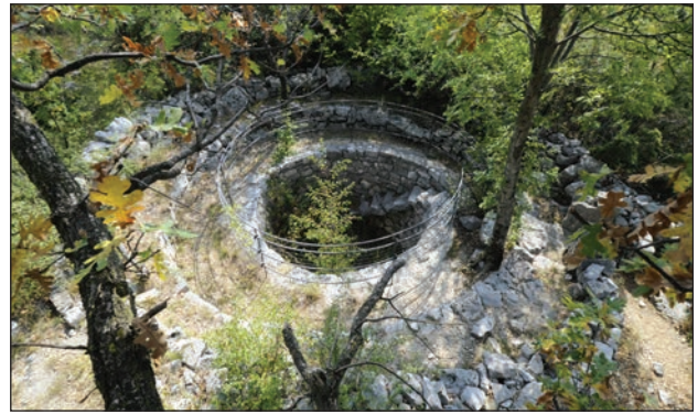
Figure 13: Lokvica in the Slovene language means ‘a small pond’: the well is about five metres deep, but in 2012 was without any water (Photo: B. Juvanec).
