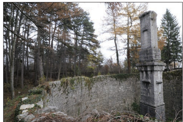
Figure 19: Kačiče icehouse has a magnificent column in the middle, as a support for the cone-shaped carpentry roof, covered with clay tiles. The icehouse was in use in the sixties of the last century, today it exists only as a relic of the former successful economic activity (Slovenia) (Photo: B. Juvanec).
