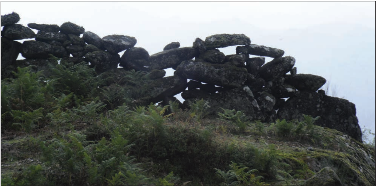
Figure 4: This incredible type of wall in single construction, called a 'unjulica' (single wall), on the island of Cres separates flocks and protects them from unsafe areas. It is permeable but also resistant against strong winds. It doesn't use a lot of material for a massive construction, which cannot be found there (Photo: B. Juvanec).
